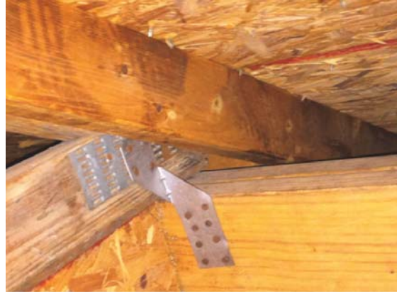
Hurricane clip roof to wall attachment
