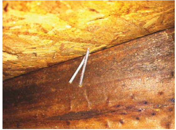
Type A roof deck attachment
