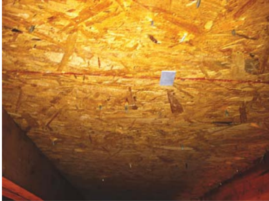
Six nails per shingle from roof underside
