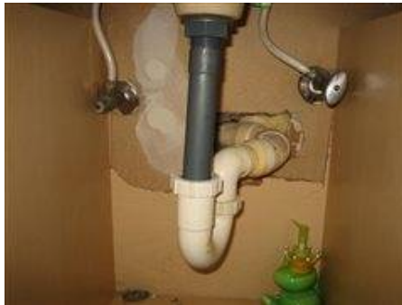
Photo 26 Under bathroom sink 1
