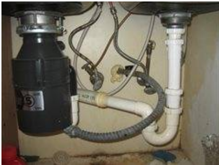
Photo 21 Under kitchen sink
